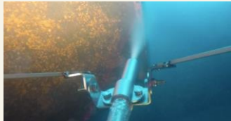
Spot Cleaning of Marine Growth
