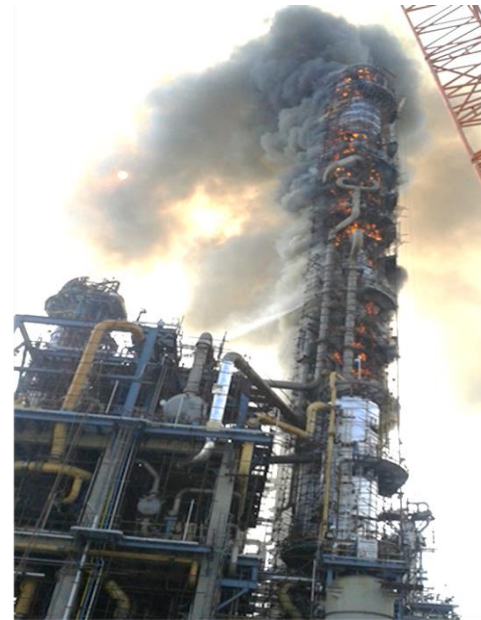
Isomerization reactor certified by TCR with detailed FFS Study post-Fire damage
