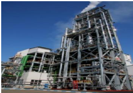
Equipment operating in creep range and cyclic services
