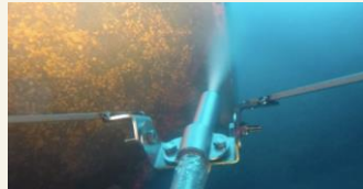
Spot Cleaning of Marine Growth
