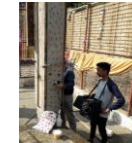
UPV Testing on column
