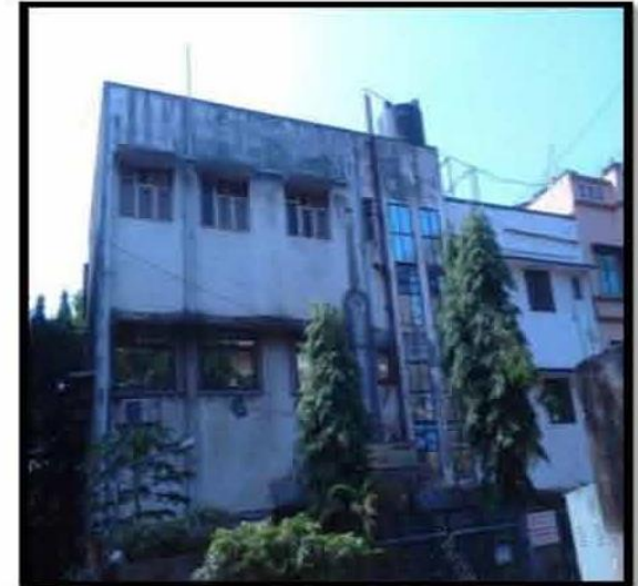
Essential Power transmission Pvt. Ltd., Andheri (Corporate building)
